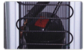
Hermetically sealed reciprocating Compressor
